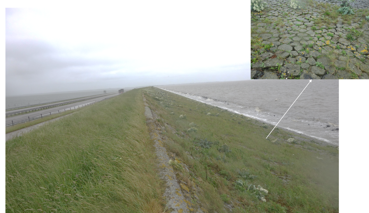
Seaside slope viewing North of Afsluitdijk
