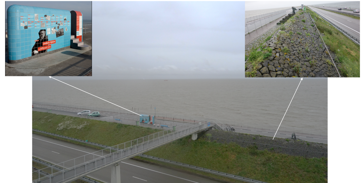
The Monument location at the middle. On the top left the blue structure showing the history of the Afsluitdijk. On the right showing the basalt revetment near the statue.
