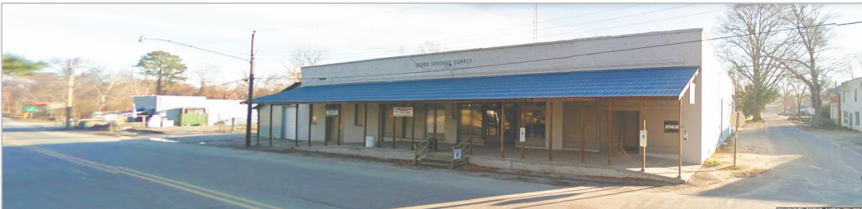
Existing Tidewater Building.
