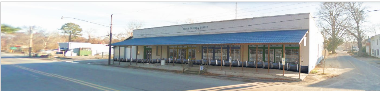
Tidewater Building protected by both wet flood-proofing (elevate interior first floor) and dry flood-proofing exterior with a rapid deploying, screen-mesh product.
