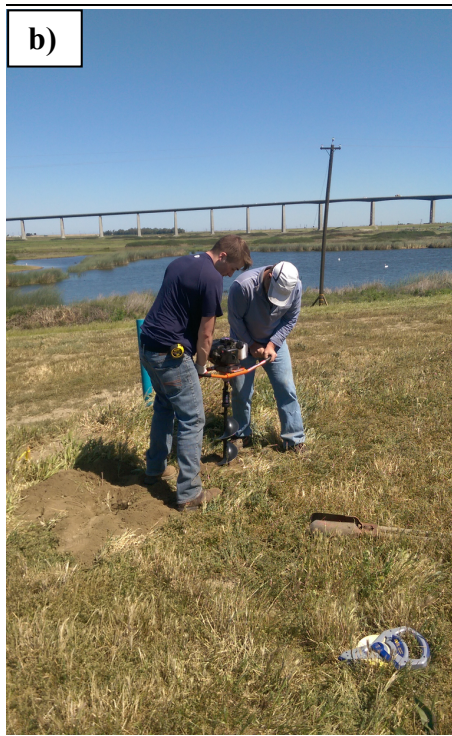
Figure 1. a) Location of in situ GPS stations (approximate coordinates: 38^{\circ}01'56.81'' N, 121^{\circ}45'49.09'' W); b) Installation of pedestal foundation for GPS station; c) completed autonomous GPS station (8003).
