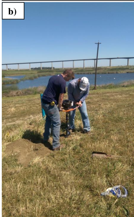
Figure 1. a) Location of in situ GPS stations (approximate coordinates: 38°01'56.81" N, 121°45'49.09" W); b) Installation of pedestal foundation for GPS station; c) completed autonomous GPS station (8003).
